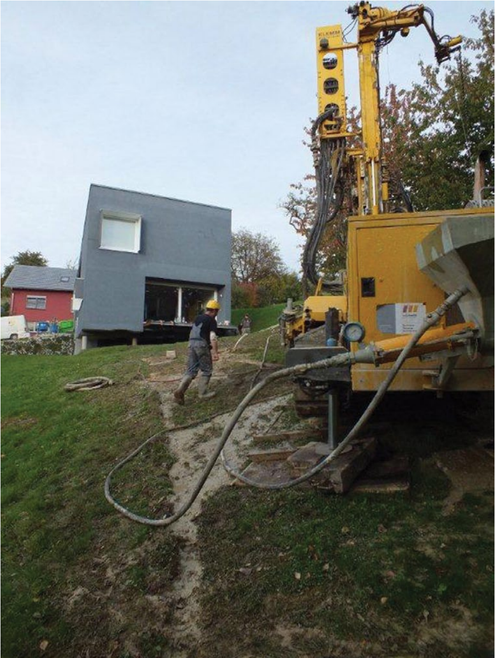
10 Drilling equipment for installation of the ground source heat pump
